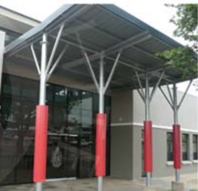
Kokstad Municipal Offices
