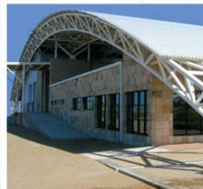
ELIDZ Container Yard
